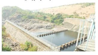
Downstream side of Watrak Dam with Energy Dissipators
