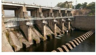
Ogee type Spillway at Watrak Dam
