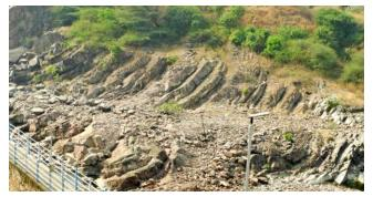
Erosion on Downstream side due to Overflow of water from Spillway Section
