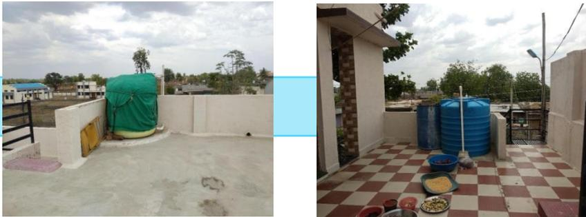
**Figure: 1 Elevated water tanks (a) 1000 litres on first floor slab (b) 700 litres on ground floor slab.**
