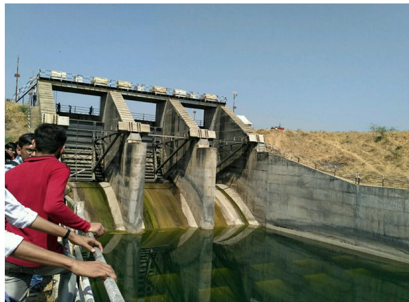
Sabarmati Escape Structure with 3 nos of Radial Gates
