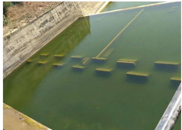
Energy Dissipators at Downstream side of Sabarmati Escape Structure
