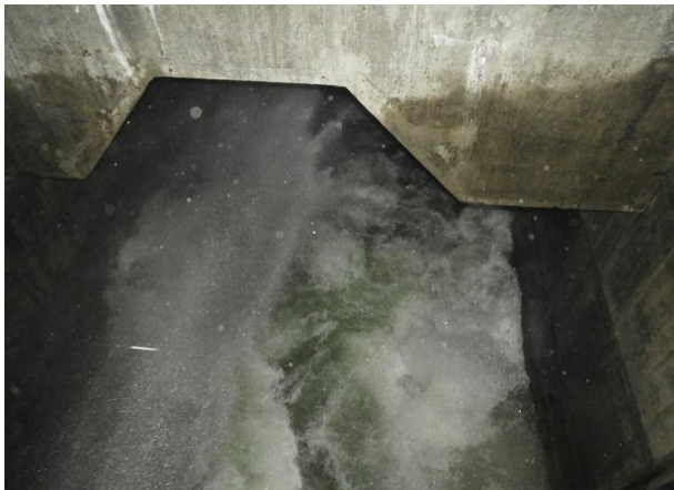
Water entering Sabarmati Canal Syphon
