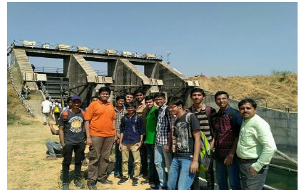
Downstream side of Sabarmati Escape Structure
