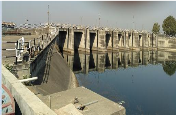
View of Sabarmati Canal Syphon from Upstream Side
