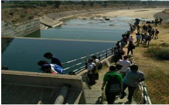
Tail Canal at Downstream side of Sabarmati Escape Structure
